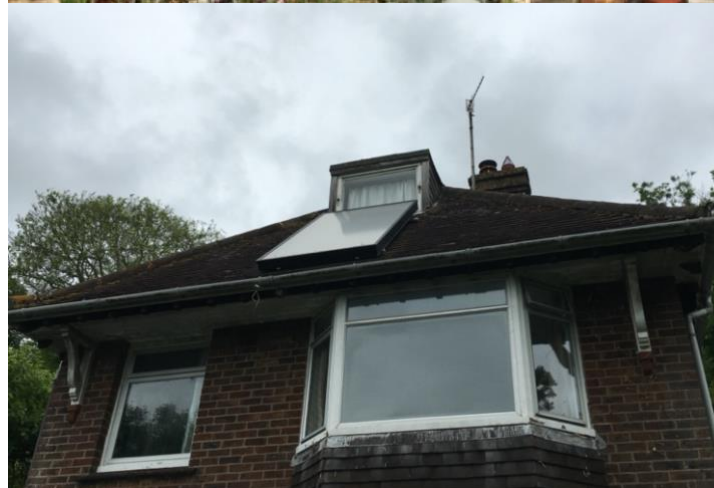
(Benallan front dormer – hanging tiled bay below)
