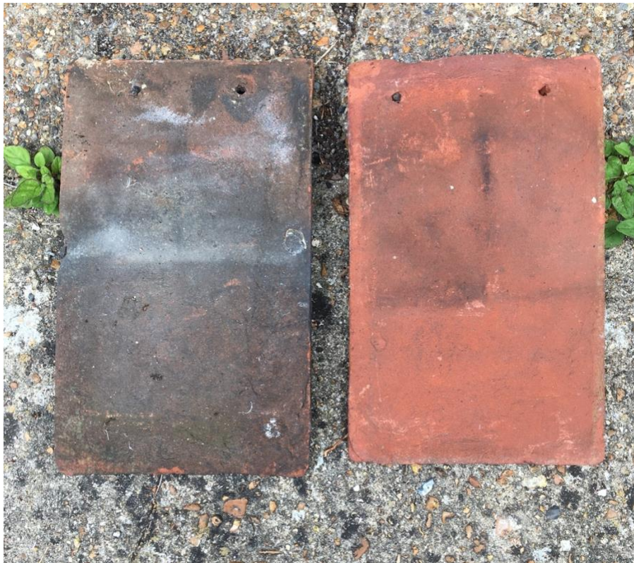
(Existing spare hanging tiles from the house)
